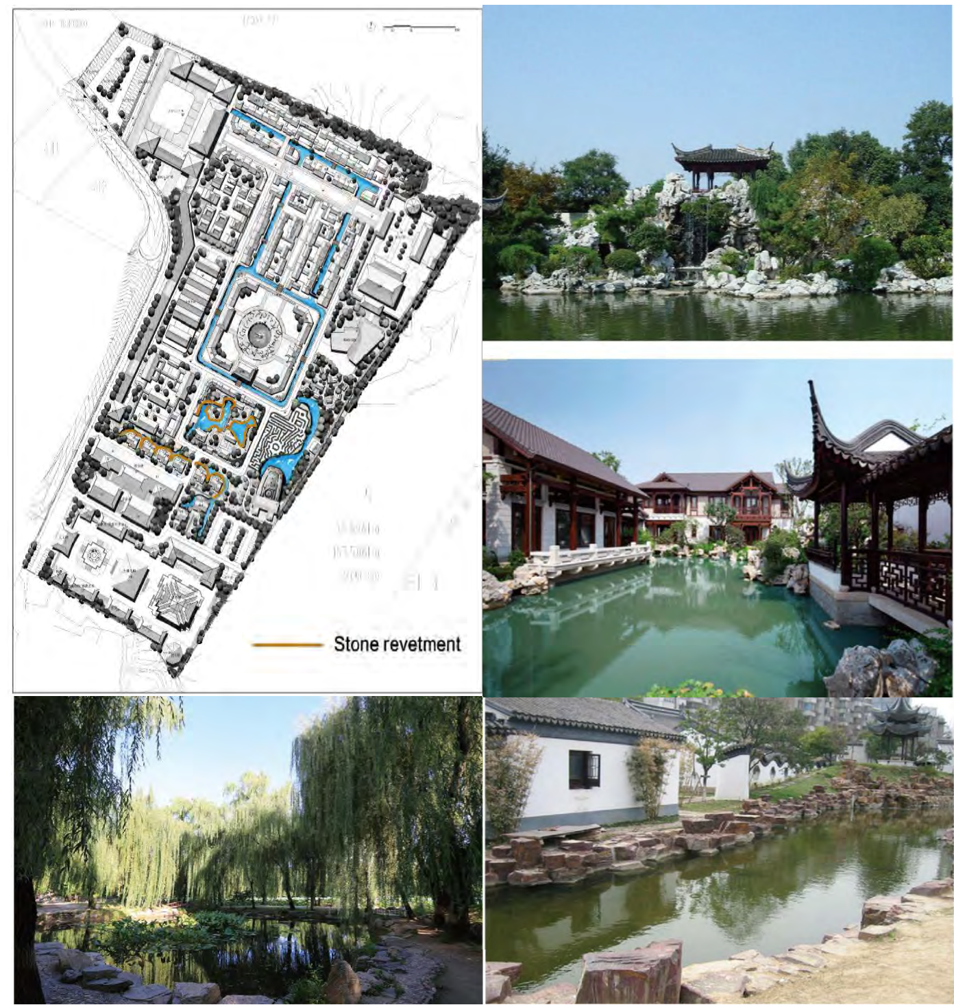
Natural stone / Contoured Naturalistic, sculptural edge using carefully selected and placed stone and rock pieces. Allows close access to water bodies and provides opportunities to use stone as a sculptural element in the tradition of Chinese landscape design.
